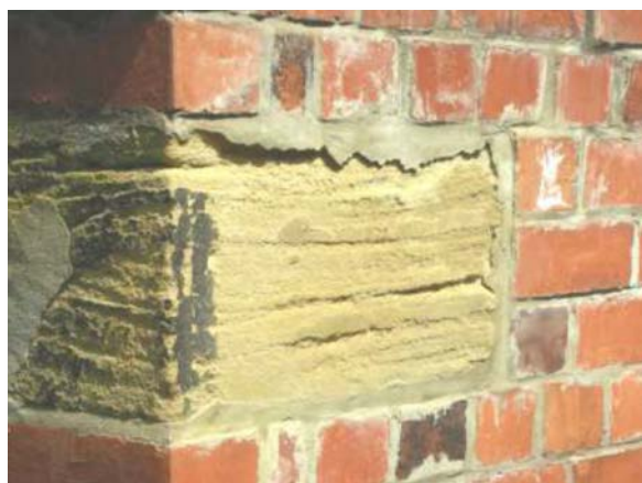
Bolton Road – stone erosion caused by inappropriate and poor repointing
