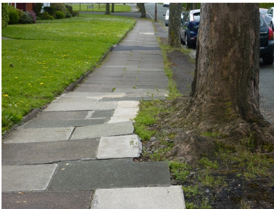
Pool Bank – uneven paving caused by root upheaval
