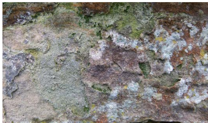
Balustrade – the top course of stone in the retaining wall exhibits heavy biological growth and salt deposits, causing the surface of the sandstone to blister and detach
