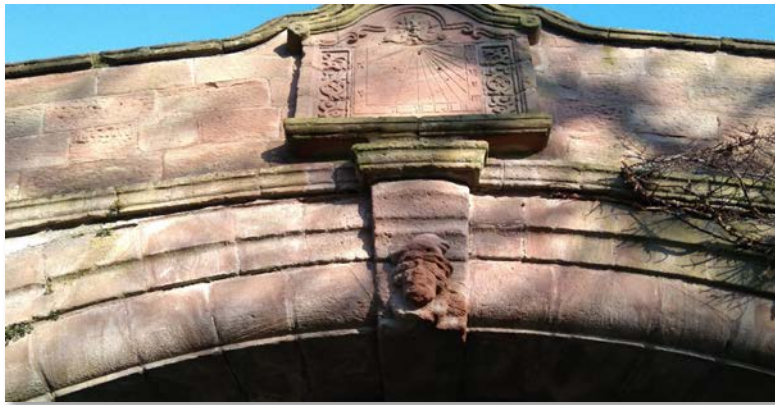
The Dell Bridge – carved ornamental detail at the busts is highly eroded and legibility has been lost. Elements of the sundial are also missing.
