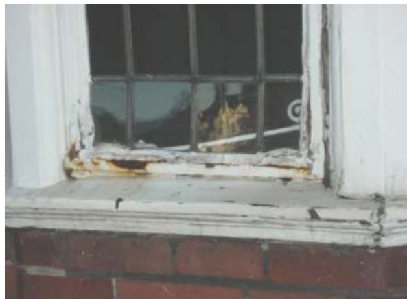
New Chester Rd – rusting metal casement window
