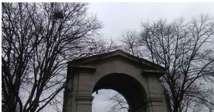
Mature trees overhang the arch – leaf/branch drop and shade may contribute to the deterioration of this Portland stone site
