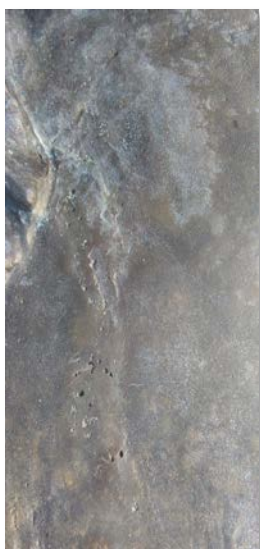
A specialist bronze conservator will be required to investigate pitting and minor pustules on the Leverhulme Memorial
