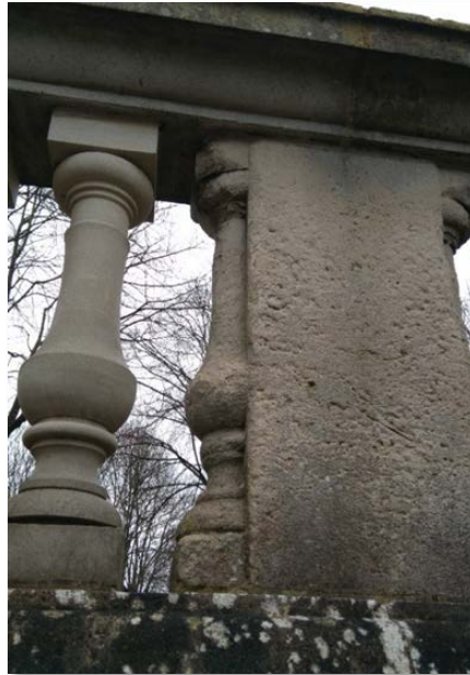
Previous abrasive cleaning of the balustrade appears to have damaged the surface of the Portland stone (which initially had a smooth finish)
