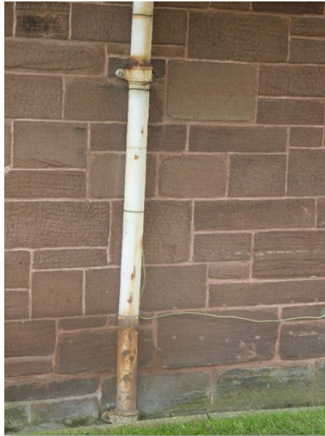
Bebington Rd – rusted downpipe in need of repair
