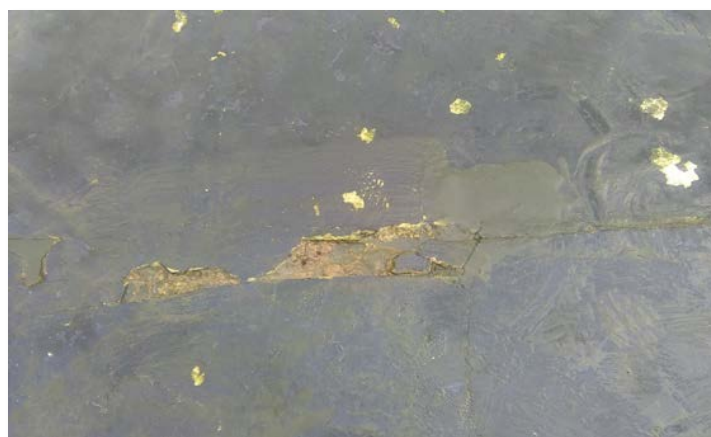
The base of the boating pond is cracked extensively, and sections of screed are missing/detached
