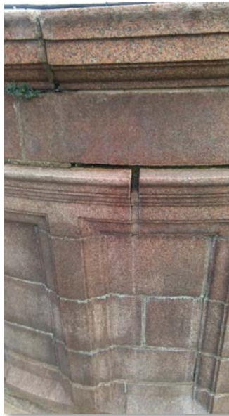
Widespread loss of pointing mortar has resulted in deep and often wide-open joints at the Silver Wedding Anniversary Fountain
